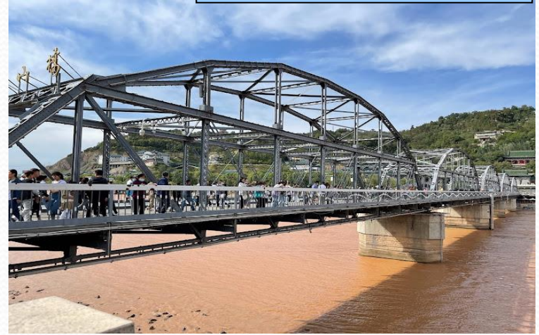
Yellow River Bridge
