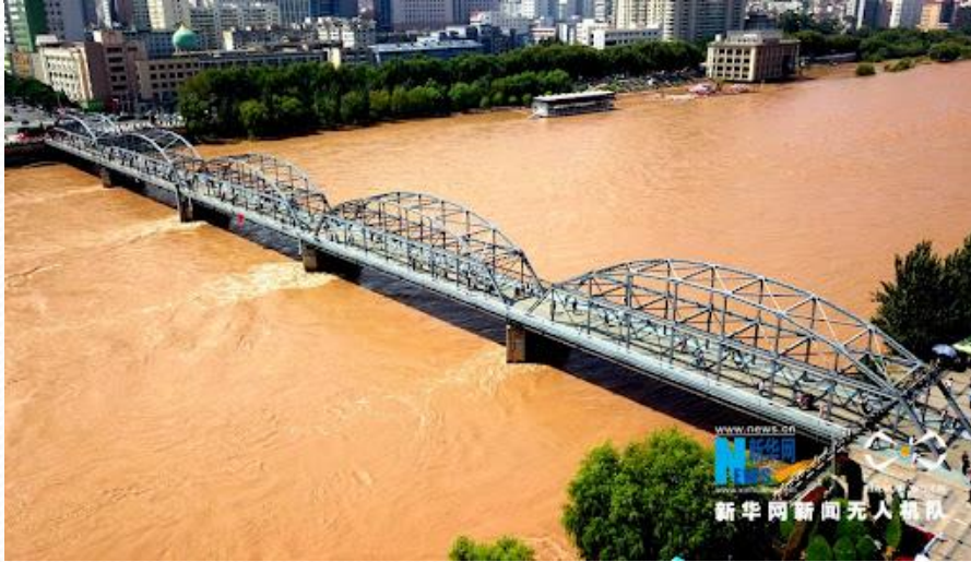
Yellow River Bridge
